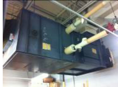
Typical Air Handling Unit
