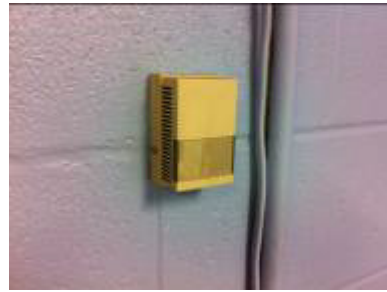
Typical Pneumatic Thermostat
