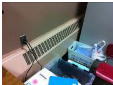
Typical Fintube Radiation
