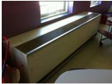
Typical Unit Ventilator
