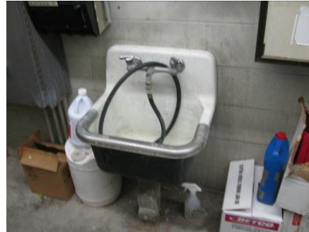
Typical Janitor's Sink
