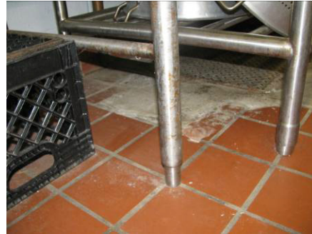
Grease Interceptor Recessed in Floor
