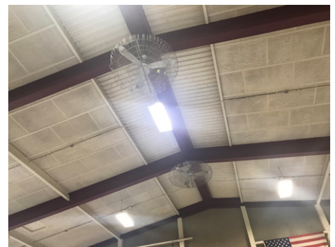
Existing Gym Destratification Fans
