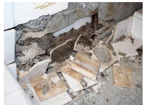
Damaged tile walls in Locker Rooms
