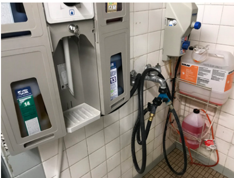
Janitor's Sink with Chemical Dispenser
