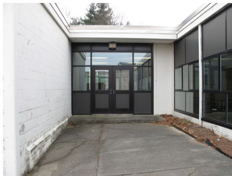
Courtyard view of non-compliant building access
