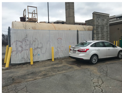
Existing 10,000 Above Ground Oil Tank
