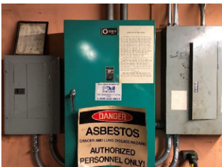
100A Transfer Switch
