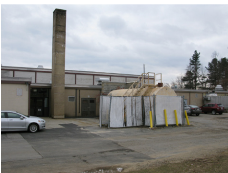
View of rear of building
