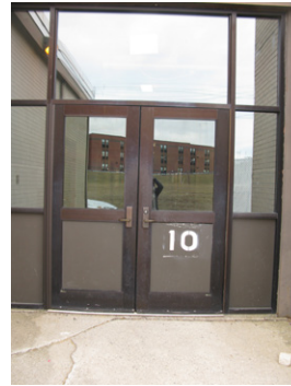
View at secondary entry
