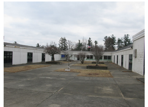
View of court yard
