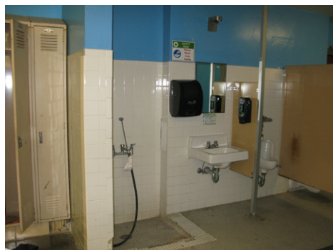
Non-compliant custodial sink. Damages wall/floor tile and plumbing fixtures
