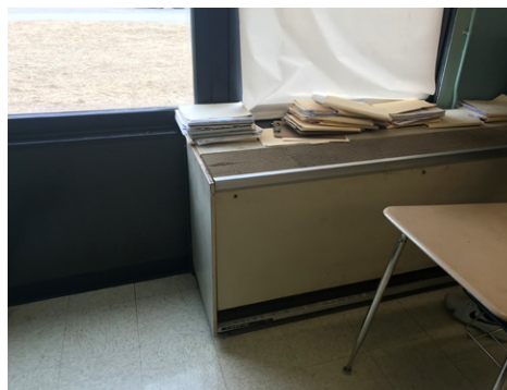
Existing Classroom Unit Ventilation and Fintube Radiator
