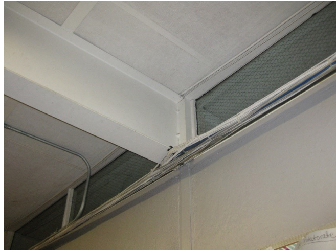
PHOTO 4: Roof beam bearing on interior column with concrete wall panels below clerestory windows
