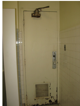
Non-compliant door clearances
