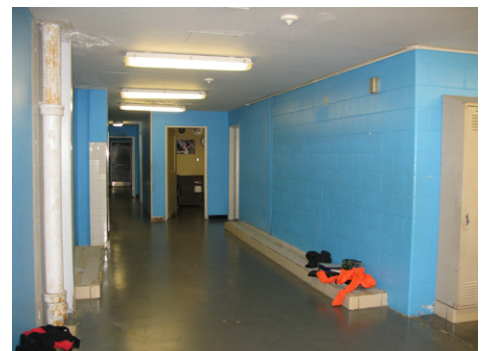
No lockers in Locker Rooms
