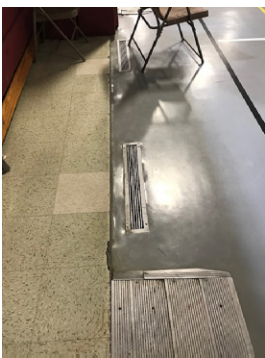
Existing Gym Air Outlet
