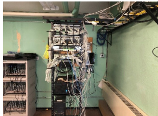
Main Communications Rack
