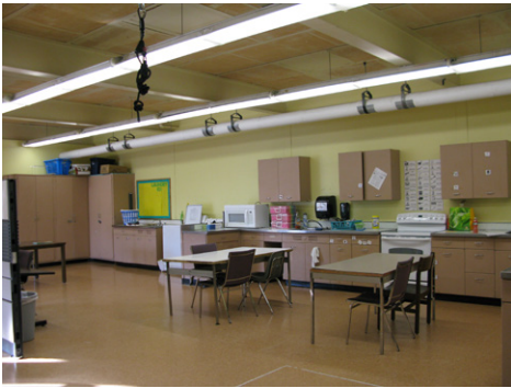
Non-compliant sinks, cabinets and clearances in Life Learning Classroom
