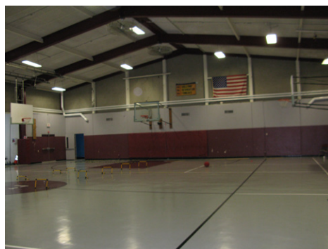
Undersized gymnasium with inadequate seating and spectator area
