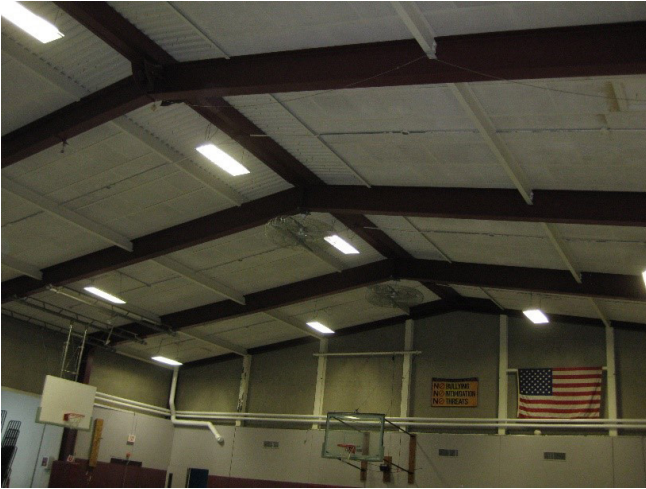
PHOTO 3: Steel roof bents in gymnasium
