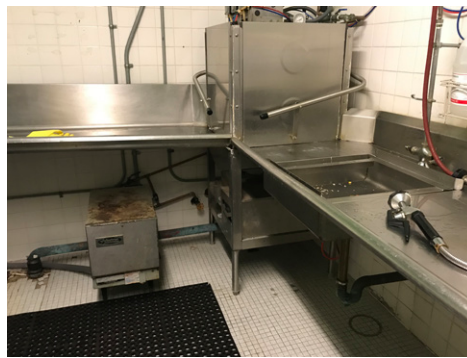
Electric Hot Water Booster at Dish Machine
