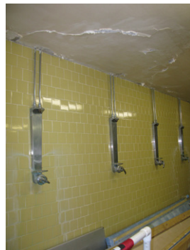
Non-compliant showers/water damaged ceiling
