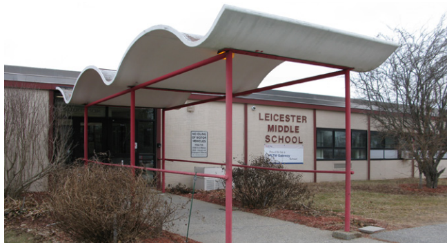
View at Main Entrance
