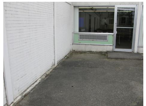
Courtyard view of non-compliant Library access
