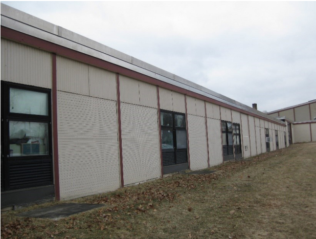
PHOTO 5: View from exterior showing exterior steel columns and steel channel at roof line (painted in red).
