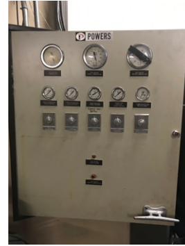
Defunct Water Heater
