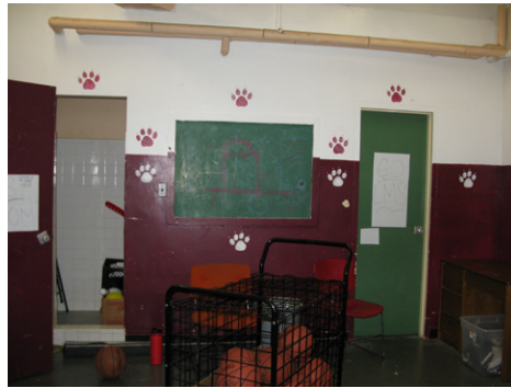
Team Locker room with non-compliant shower and bathroom
