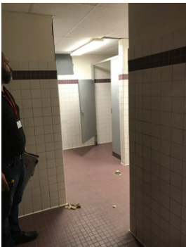
Partial accessible bathrooms
