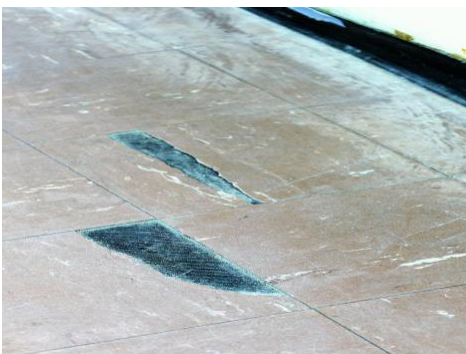
Damaged and worn flooring finishes
