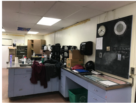
Non-compliant sinks, cabinets and clearances in Science Classrooms
