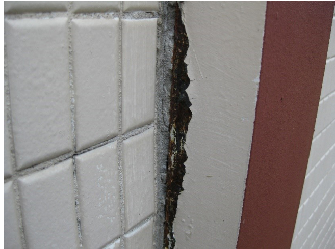
Photo 6: Close up of column showing slight rusting of steel
