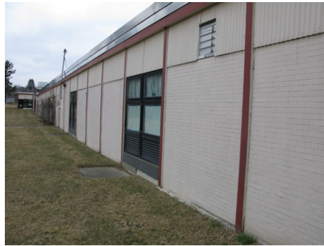
View of exterior wall assembly
