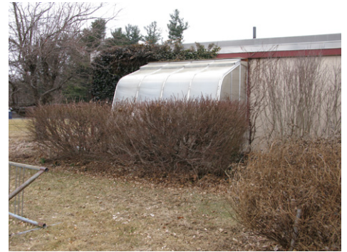
View of greenhouse
