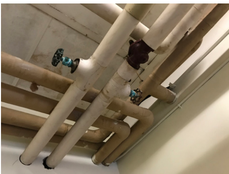
Existing Hot Water Piping
