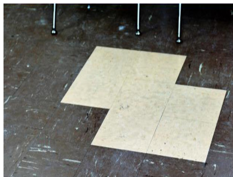
Poor patching of existing finishes
