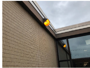
Exterior Sodium Vapor Lighting
