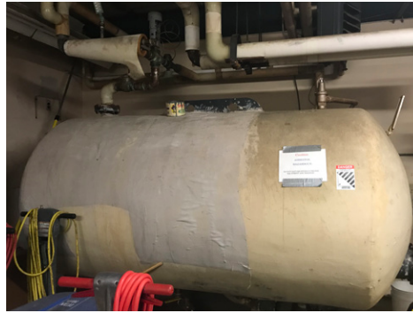
Domestic Hot Water Storage Tank
