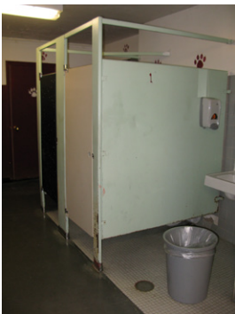
Non-compliant locker room toilets
