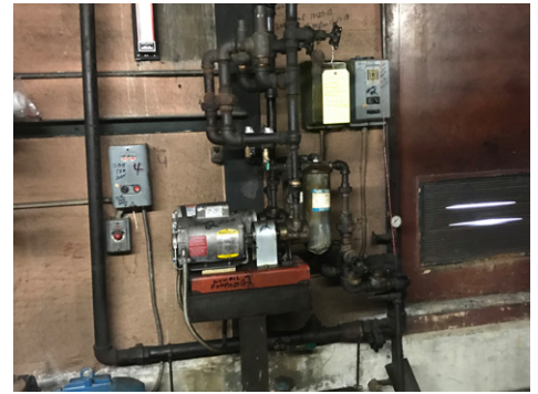
Existing Fuel Oil Pump
