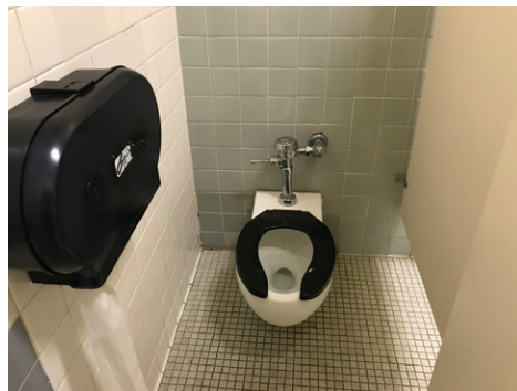
Typical Plumbing Fixtures 3
