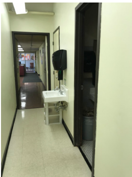
Non-compliant sink/clearances in corridor
