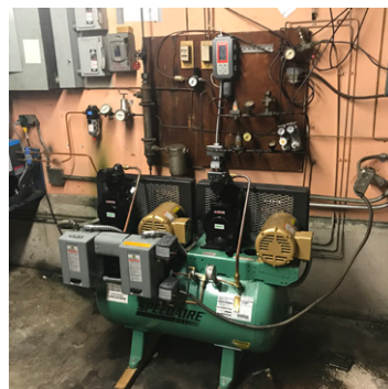
Existing ATC Air Compressor
