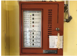
Fire Alarm Panel
