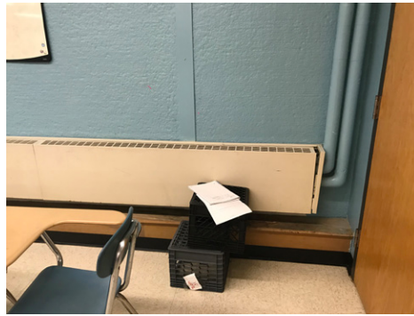
Existing Fintube Radiator
