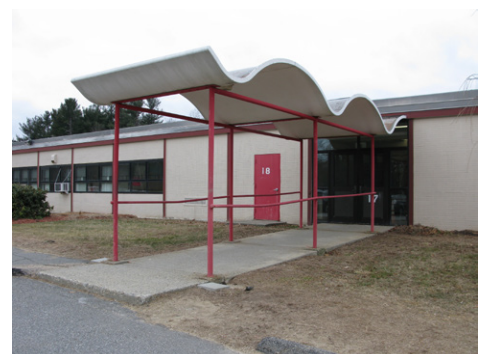
View of non-compliant Main Entrance building access
