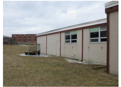
View of West Elevation towards playing fields
