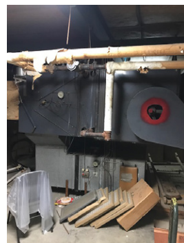
Existing Heating Ventilating Unit
