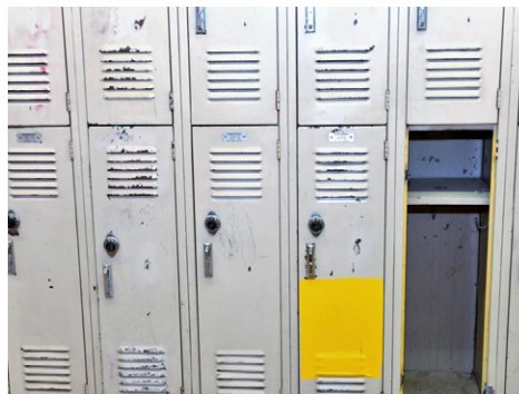
Damaged and inoperable lockers
