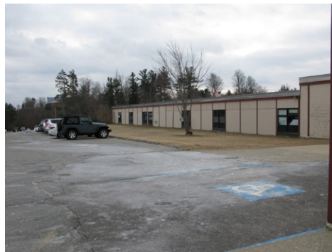
View of main parking lot
