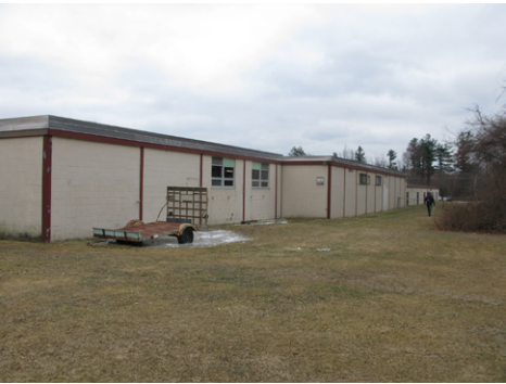
View of North West Elevation from playing fields
