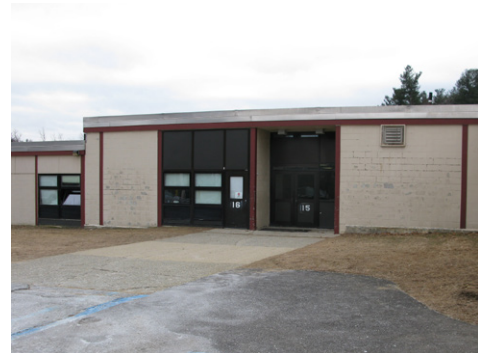
View of East Entrance from main parking lot
