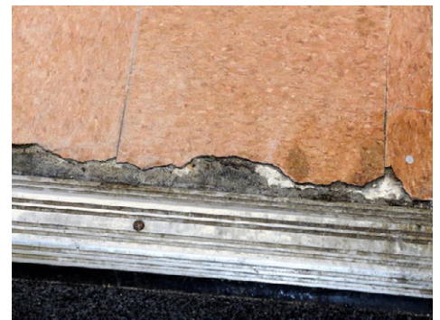
Damaged flooring at material transitions
