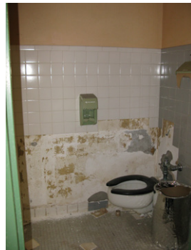
Deteriorated wall tile
