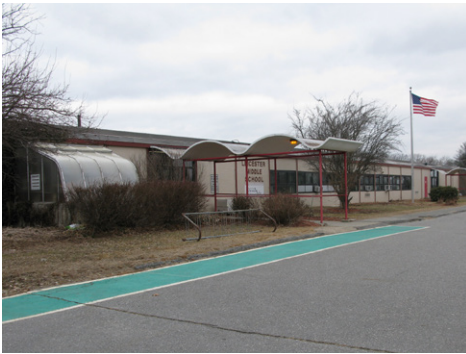
View of Main Entrance
