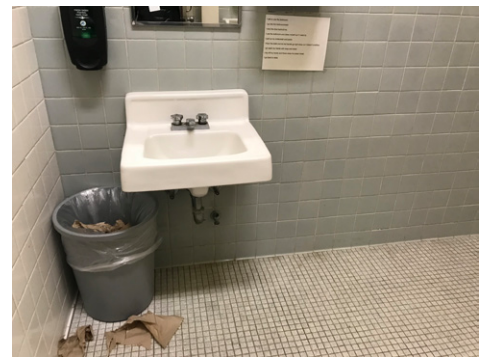
Typical Plumbing Fixtures
