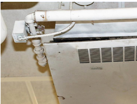
Retrofit mechanical equipment
