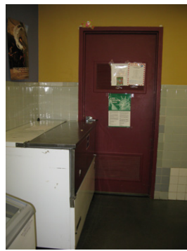
Non-compliant door clearance in server
