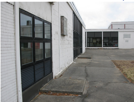
Courtyard view of non-compliant access
