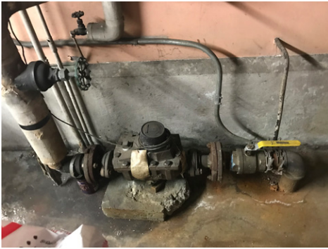
Domestic Water Service
