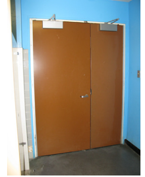
Non-compliant doorswing direction
