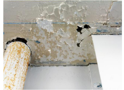
Water damaged plaster and paint
