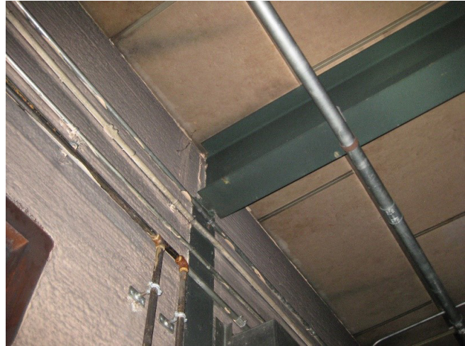
PHOTO 1: Interior beam framing into steel column. Concrete wall panel nested between column flanges.
