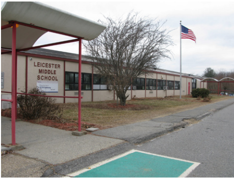
Non-compliant main entrance
