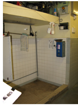
Non-compliant custodial slop sink in kitchen
