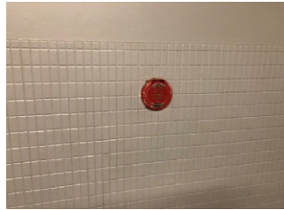
Noncompliant Pull Station
