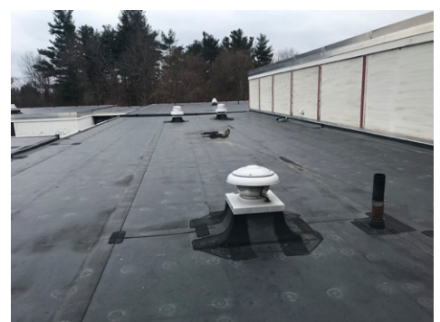
Existing Roof Top Equipment
