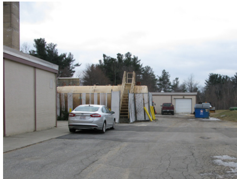
View of propane storage tank at rear
