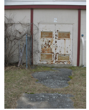
Exterior mechanical room access
