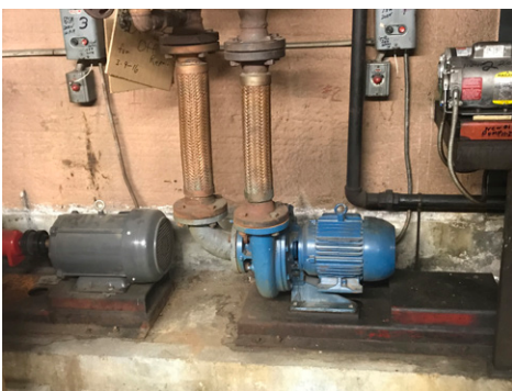
Existing Hot water Circulating Pumps
