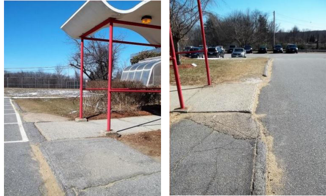
Non-compliant Main Entrances
