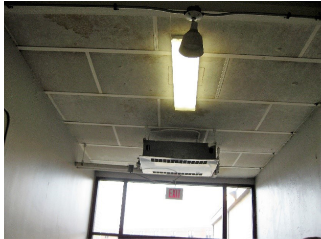
PHOTO 2: Minor water staining of gypsum roof panels
