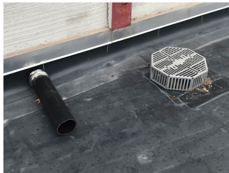
Insert Type Roof Drain
