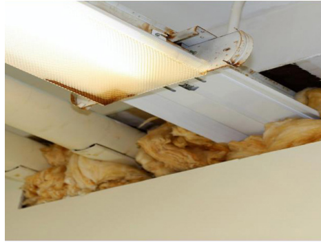
Light fixture penetrating stud wall
