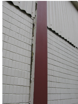
View of corrugated plastic, failing tile & rusted steel
