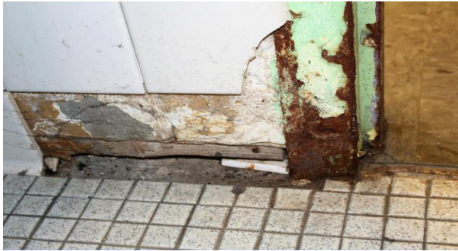
View of wall deterioration on Locker Rooms
