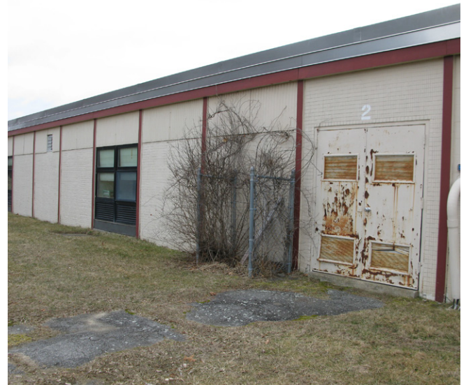
View at West Elevation
