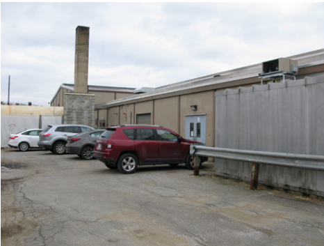
Service entrance for Kitchen and walk-in
