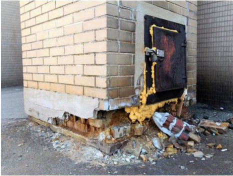
Masonry deterioration at chimney
