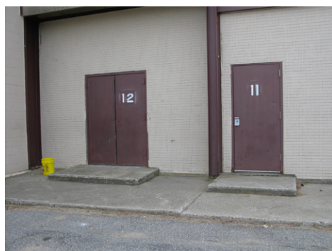
View of non-compliant building access
