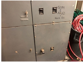
Branch Distribution Panel
