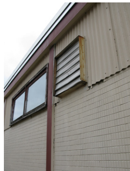
Poor condition of exterior wall assembly
