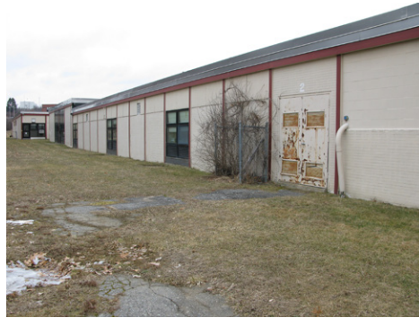
View of West Elevation
