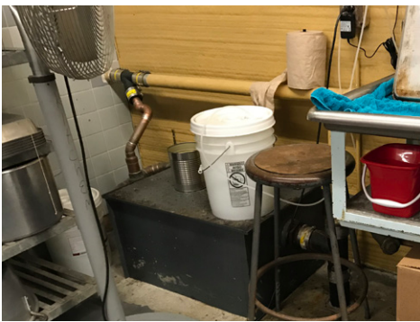
Grease Interceptor at 3-Bay Sink
