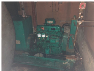
Onan 30 kW Generator
