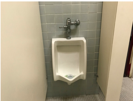
Typical Plumbing Fixtures 2
