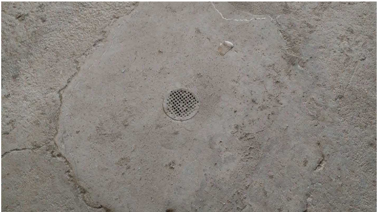
Maintenance garage floor drain.
