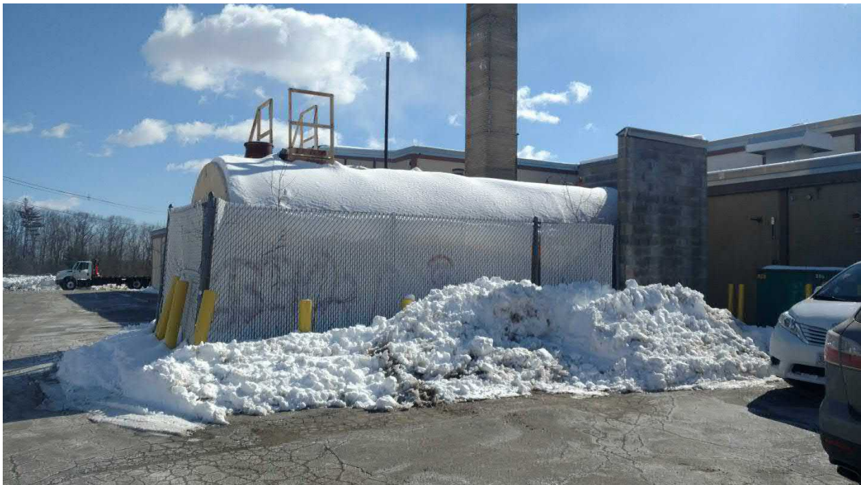
AST that fuels the boilers.
