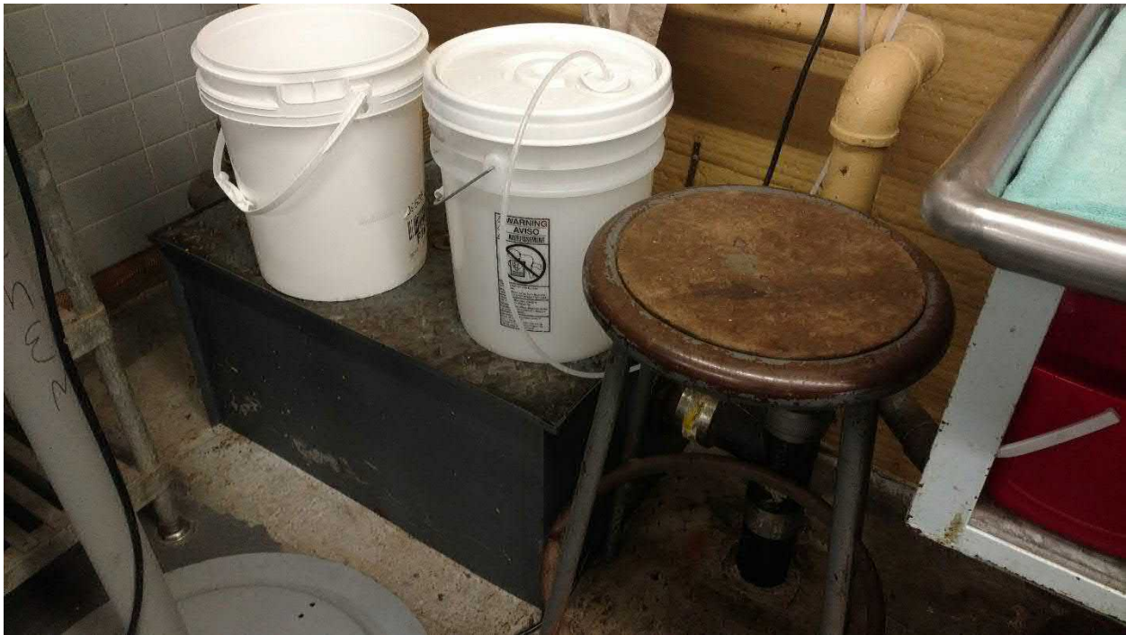
Cafeteria grease trap.
