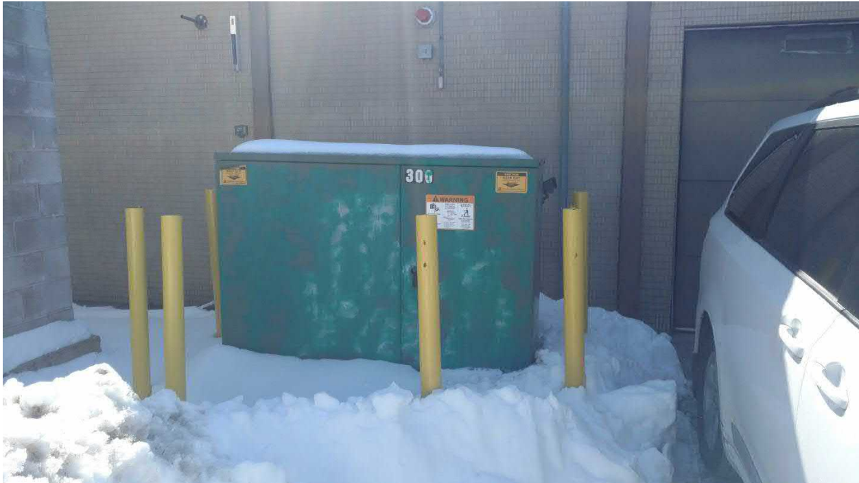
Electrical transformer.
