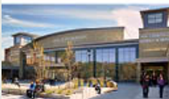
Southbridge M/H School Project Completed 7/2012 Architect: Tappe Associates CM: Consigli Construction Co. Grades: 6-12 Cost: $74M
