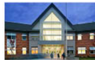
Uxbridge High School Project Completed Fall 2012 Architect: Raymond Design Associates CM: Shawmut Design & Construction Grades: 9-12 Cost: $45M
