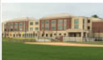
Wilmington High School Project Completed 2/2015 Architect: Dore & Whittier Associates CM: Gilbane Building Company Grades: 9-12 Cost: $83M
