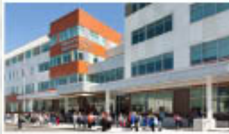
Lynn Thurgood Marshall Middle School Project Completed April 2016 Architect: Raymond Design Associates CM: Walsh Brothers Grades: 6-8 Cost: $92M
